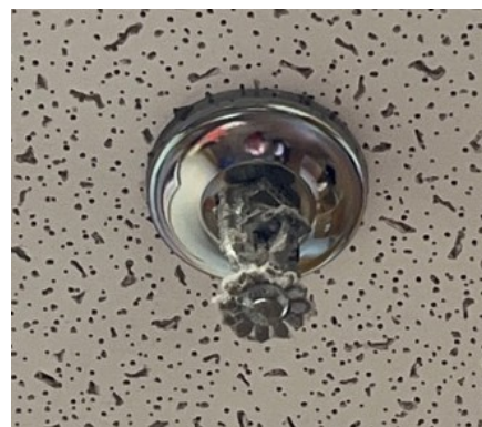
Figure B.3. Example of dust on sprinkler head noted in the emergency room at the hospital. Source: Photo taken by OIG inspector.
