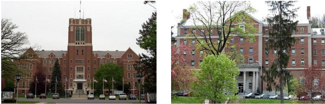
Figure 1. Canandaigua VA Medical Center (left); Bath VA Medical Center (right).
