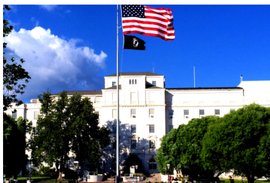
Figure 1. Bob Stump VA Medical Center. Source: "VA Northern Arizona Health Care," VA, accessed March 5, 2026, https://www.va.gov/northern-arizona-health-care .
