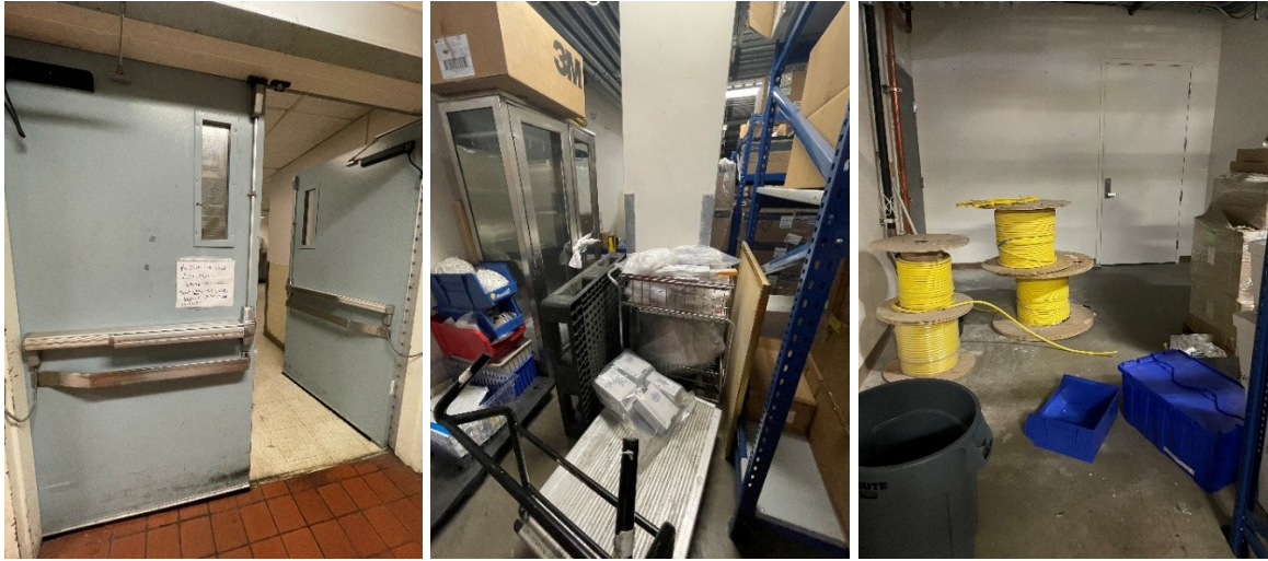
Figure 4. Entrance to the medical distribution area propped open (left) and cluttered, unclean, unmarked storage areas (middle and right) at the West Los Angeles VA Medical Center in Los Angeles, California.
